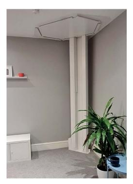
Neatly tucked away to maximise your living space, the lift guides are close the walls at each level to give you un-obstructed floor space.
