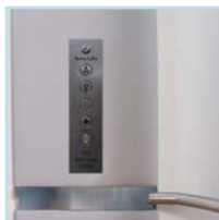
flush mounted stainless steel control console
